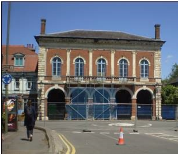
Old Town Hall, June 2018 after car accident
